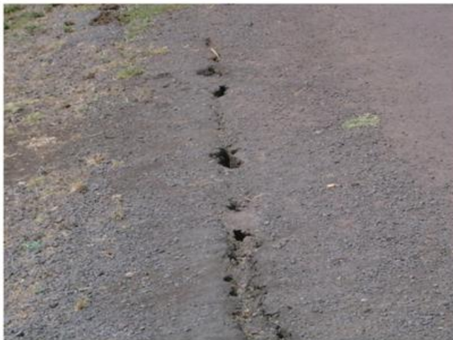
Plate 6-9 Longitudinal cracking along left side of the road (km32+150)
