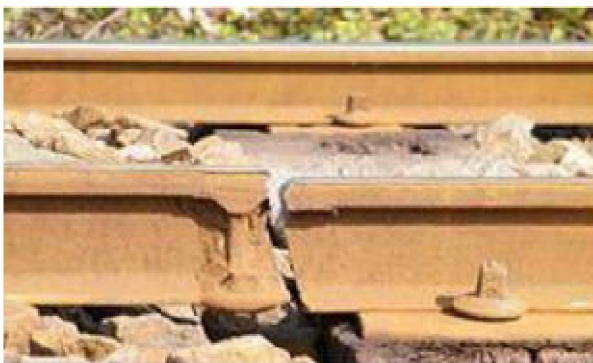
Figure 1: Crack On Railway Track
