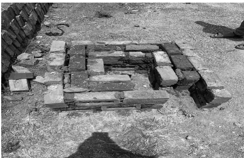
Cow dung brick in cavity wall
