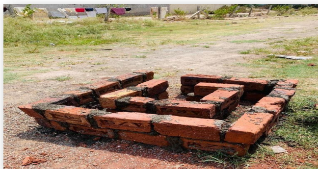
Fig 1. Structure of Cavity wall
