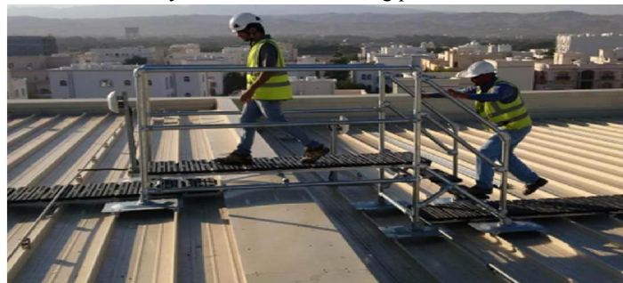
Figure 6.2: Working on Rooftop
