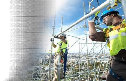
FIGER 1.1 working at elevated place
