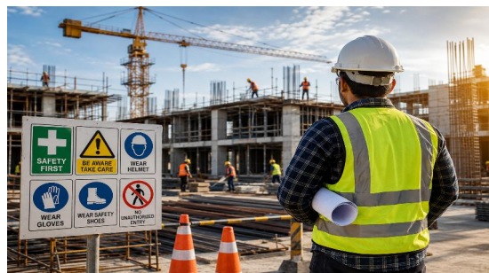
Figure: 1 Construction site
