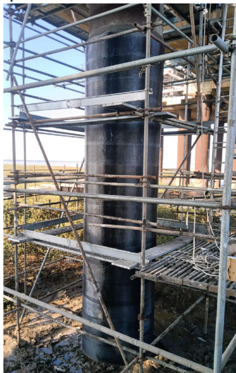
Fig 4: Application of FRP Wrapping on Bridge Pier
