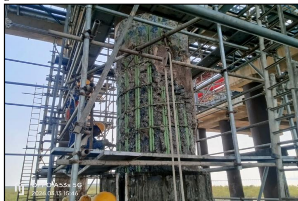
Fig 2: Damaged Bridge Pier Before Retrofitting
