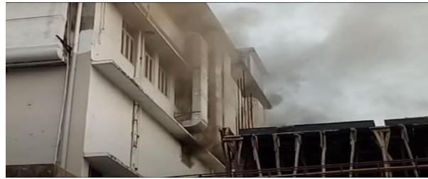
Fig 1.3 Rohini Super Specialty Hospital Fire
