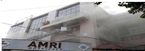
Fig 1.1 AMRI Hospital Fire
