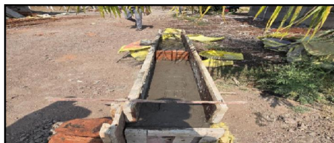
Fig.1: Casting of Reinforced Concrete Beam
