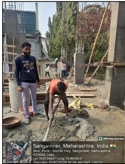
Fig 2: Concrete Mixing Stage
