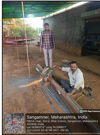
Fig 7: CFST Columns Preparation
