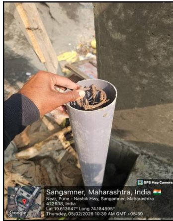
Fig 3: RC Column Preparation
