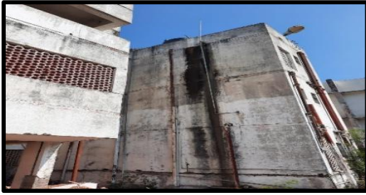
Figure 3: Crack and seepage observed.
