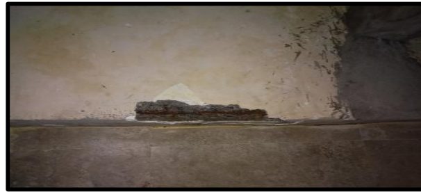
Figure 4: Reinforcement Exposed and Concrete Damage
