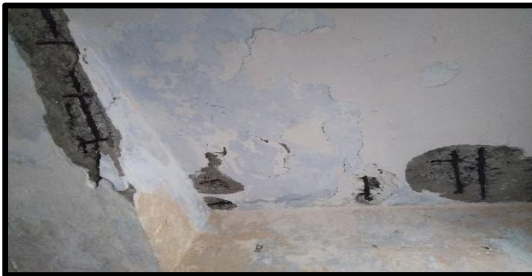
Figure 4: Reinforcement Exposed and Concrete Damage
