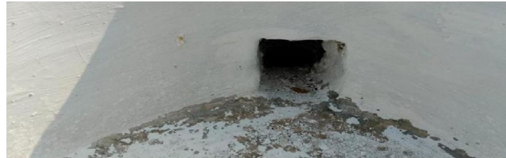
Fig No. 6.Outlet Chamber ACET Campus
