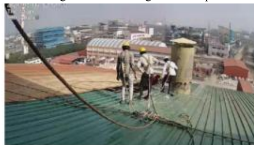
Figure 4.1: Working on Rooftop.
