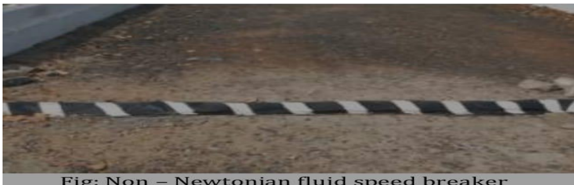
Fig: Non – Newtonian fluid speed breaker
