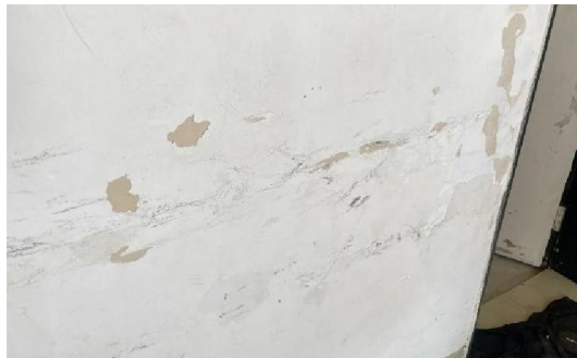
Fig. 1 – Spalling of paint
