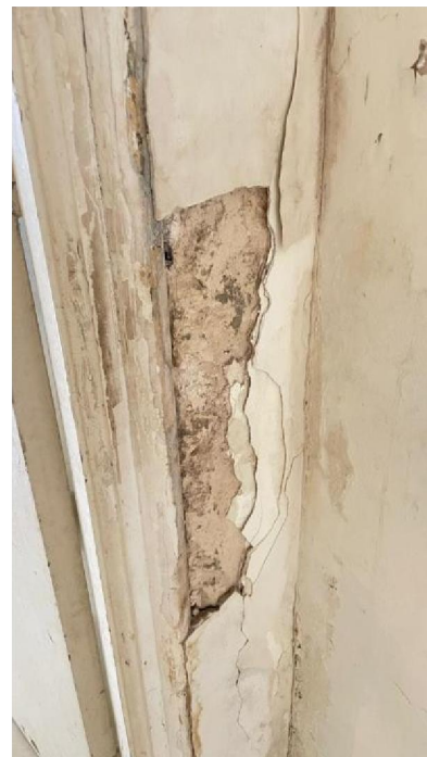
Fig. 3 – Cracks on wall
